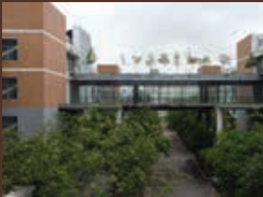
Progress Apparel, Bangladesh
